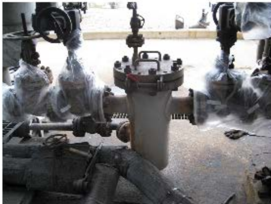
Strainer Before coating: 180^{\circ}\text{C}
