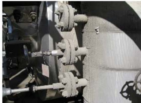
Flange After coating: 45^{\circ}\text{C}
