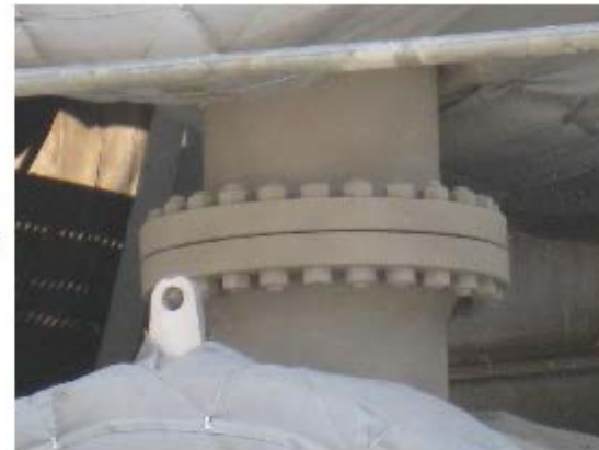
Flange After coating: 55^{\circ}\text{C}
