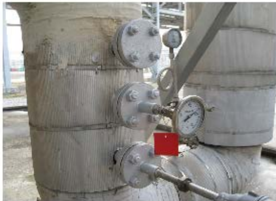
Flange Before coating: 130^{\circ}\text{C}
