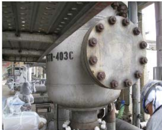
Strainer Before coating: 170^{\circ}\text{C}
