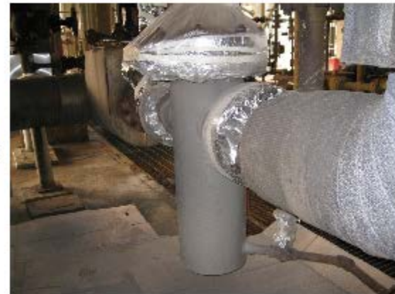
Strainer After coating: 50^{\circ}\text{C}
