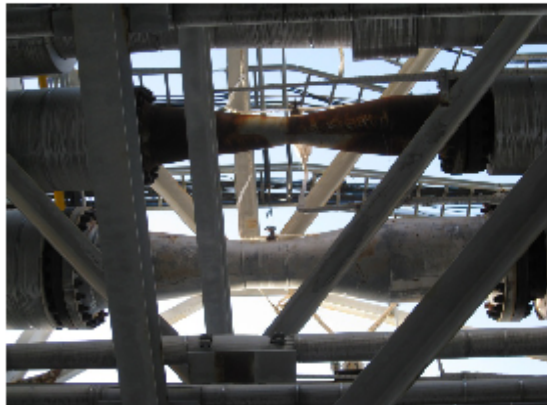
Flange Before coating: 160^{\circ}\text{C}
