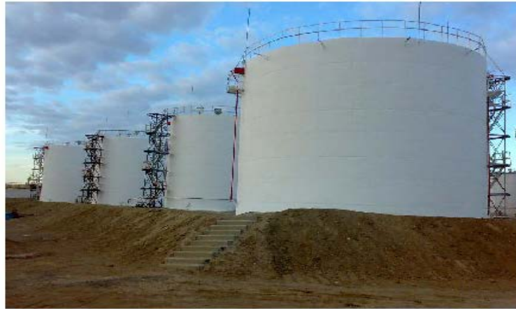
After Power Wash, RUST GRIP® and SUPER THERM®
