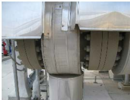
Flange After coating: 45^{\circ}\text{C}
