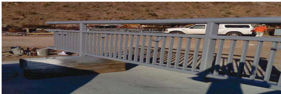
Enamo Grip topcoated Super Therm® to prevent hand oils from deteriorating surface.
