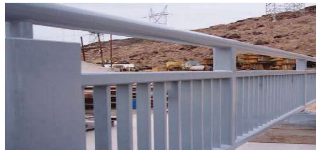
Railings were power washed at 3,500 psi and primed with Rust Grip®.
