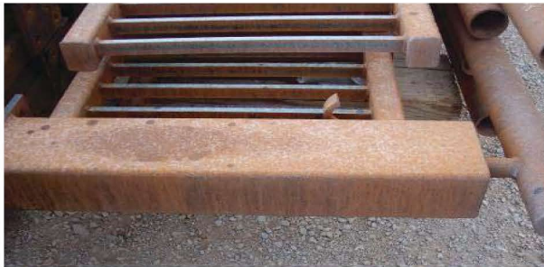
Steel railings were allowed to develop flash rust in preparation for the Rust Grip® application.
