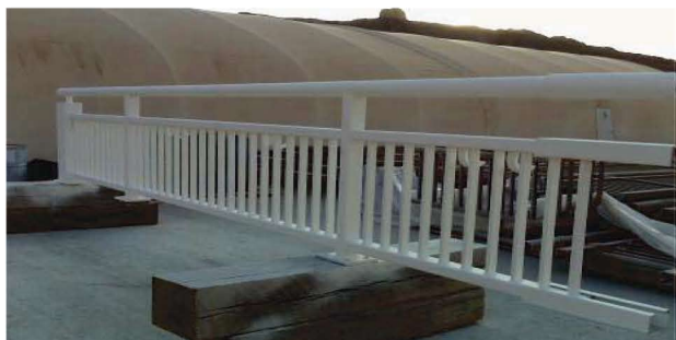
Super Therm® was applied to prevent heat from loading onto the steel railings, possibly burning visitors.
