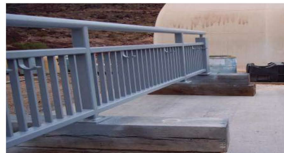
Steel railings were allowed to develop flash rust in preparation for the Rust Grip® application.
