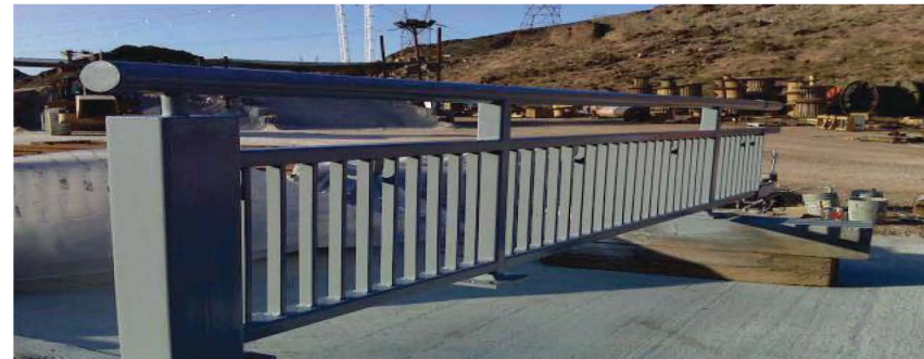
Enamo Grip topcoated Super Therm® to prevent hand oils from deteriorating surface.
