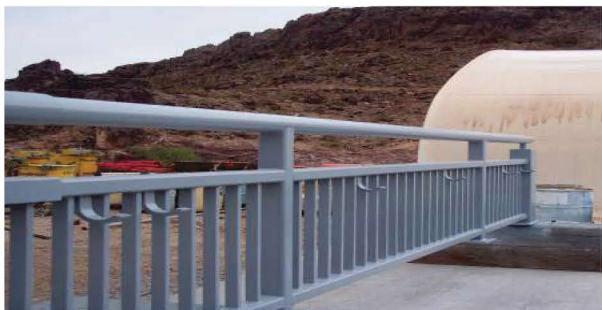
Railings were power washed at 3,500 psi and primed with Rust Grip®.
