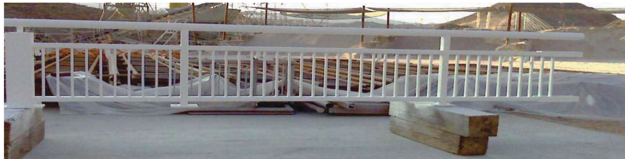
Super Therm® was applied to prevent heat from loading onto the steel railings, possibly burning visitors.
