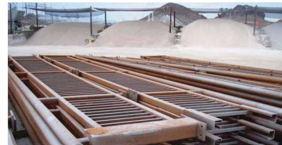
Steel railings were allowed to develop flash rust in preparation for the Rust Grip® application.
