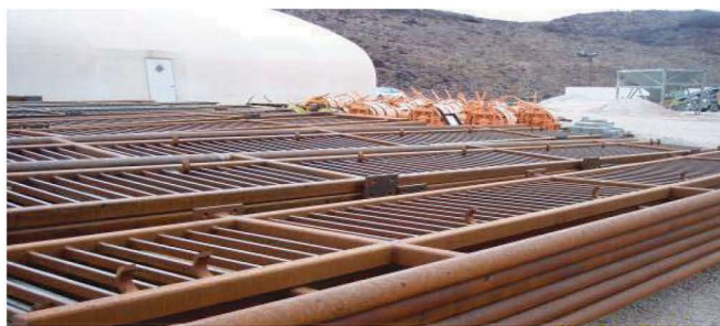
Steel railings were allowed to develop flash rust in preparation for the Rust Grip® application.
