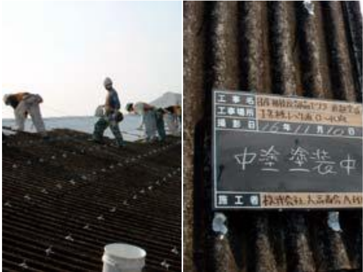
SUPER THERM ® Partially Applied
