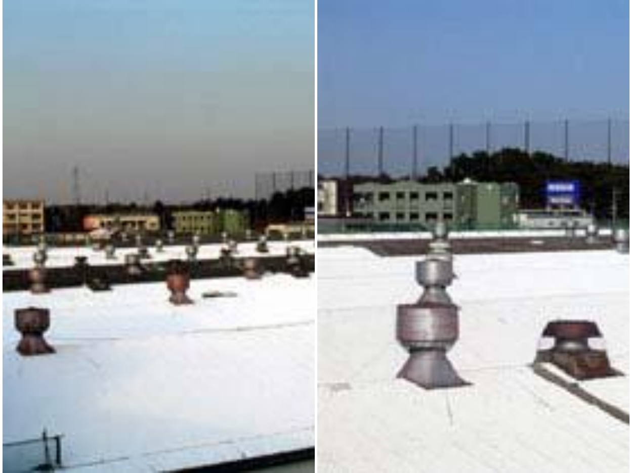
2,000,000 sq. ft. of SUPER THERM ® completely applied to the Nissan factory roof
