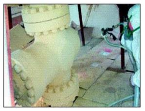
A wellhead consisting of 300mm pipes and a valve is 220C hot. The surface, which is ca. 7m2, heats up the environment and the walls of a shed, which is dome of steel and fiberglass. The heat causes damage to the fiberglass and makes work within the shed uncomfortable. The high heat also causes threat of injuries to the workers.
