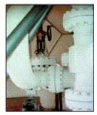
SUPER THERM is a unique combination of ceramics. Two are reflective, one acts as a dead air space between the coating surface and the substrate and the 4th blocks 99.5% infrared.
