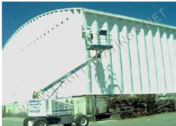
This finished system of 7 mils DFT applied in two coats, cross-hatched, provides
