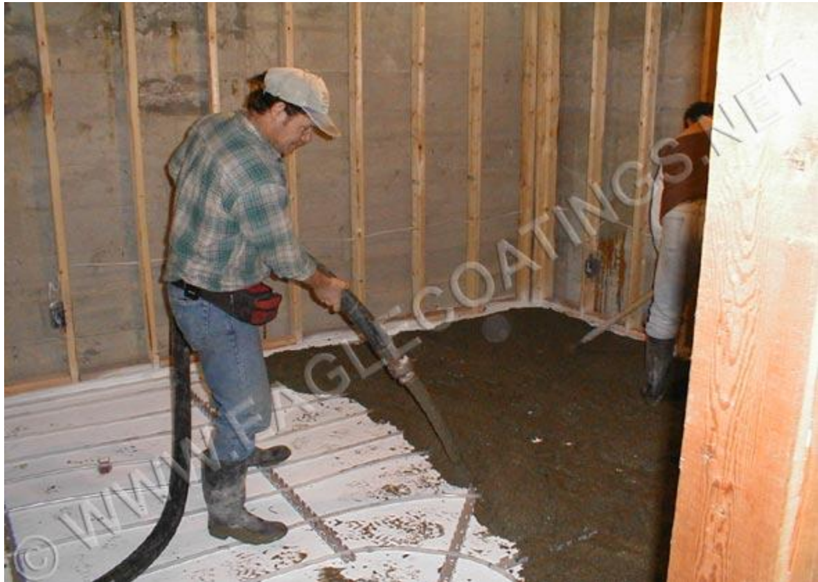
Concrete skim coat applied over entire system
