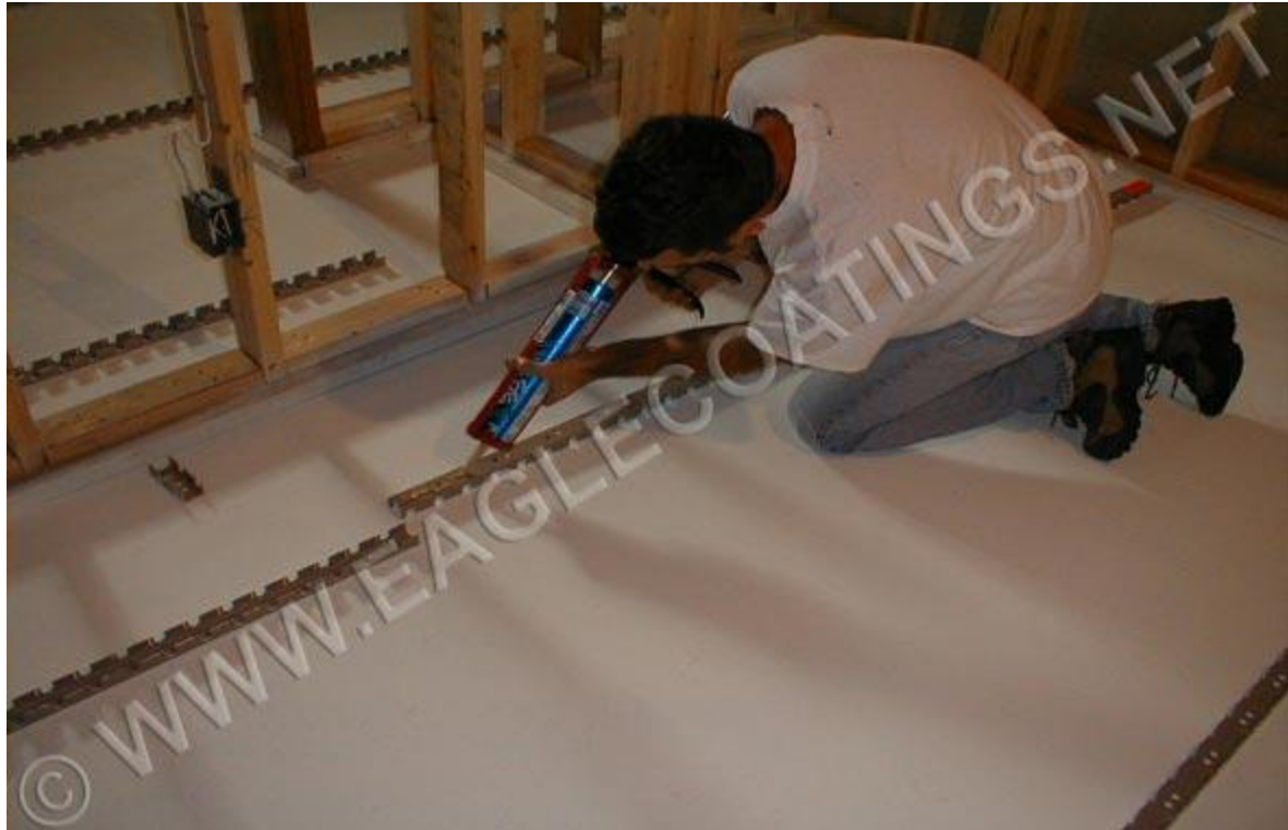
Piping rails in place
