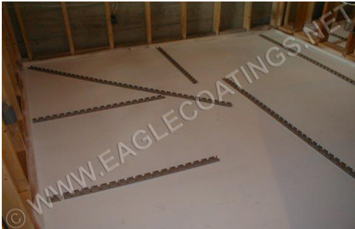
Heating tubes placed in rails
