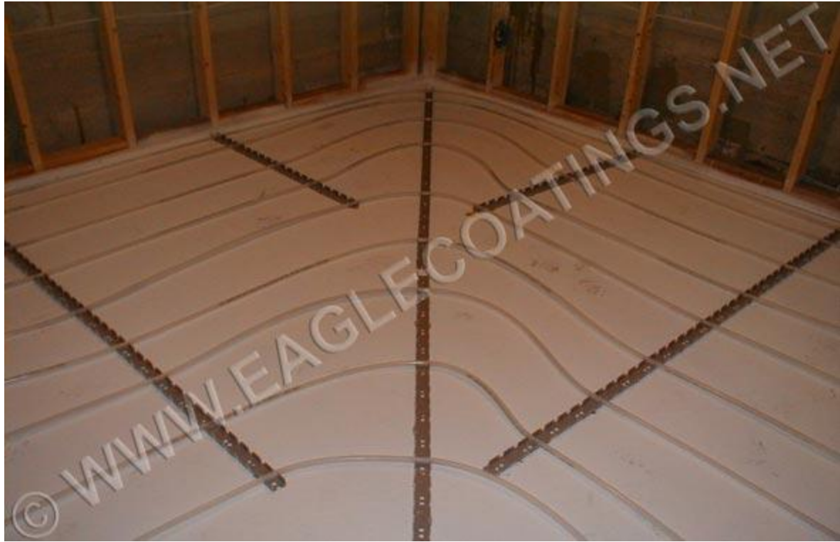
Concrete skim coat applied over entire system
