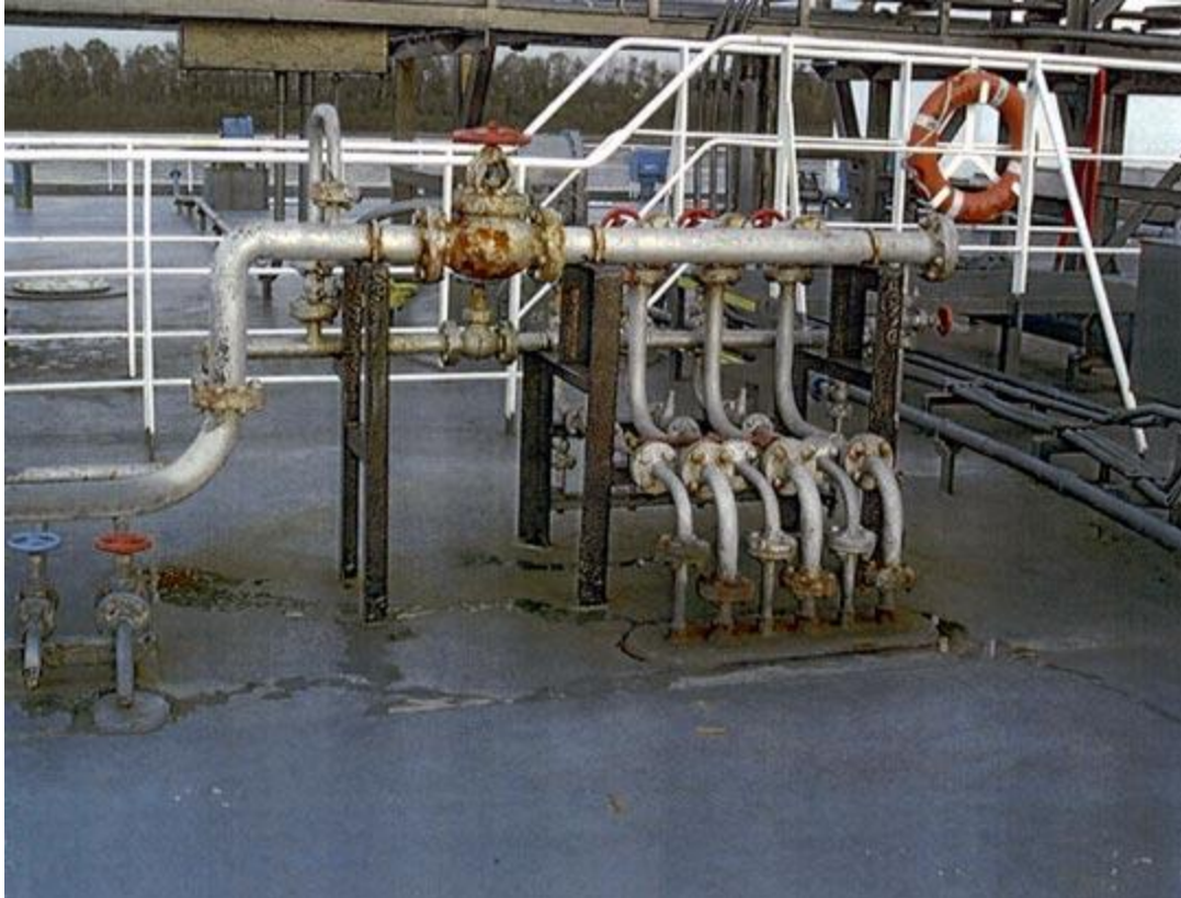
RUST GRIP® applied to Collars and Valves
