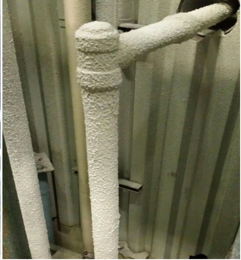
1 1/2 inch pipe 130 LF HPC ® at 14.5 mm / 571mils DFT
