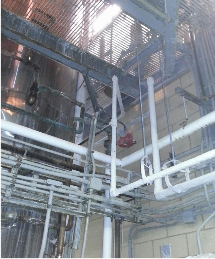
1 inch pipe 60LF HPC ® at 14 mm / 551mils DFT
