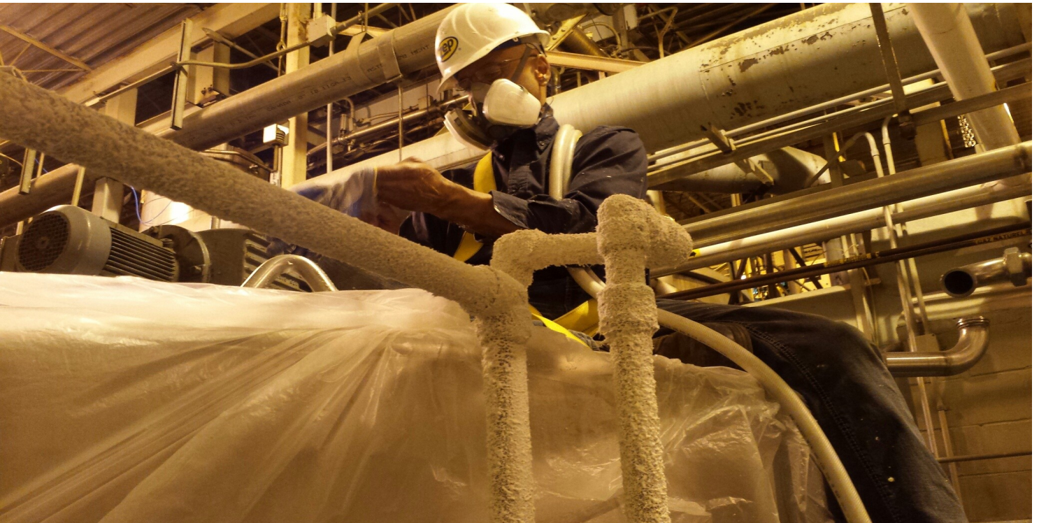
1 1/2 inch pipe 130 LF HPC ® at 14.5 mm / 571mils DFT
