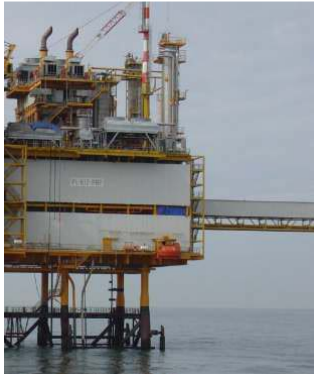
1151-B MDEA gas absorber (upper right tower)
