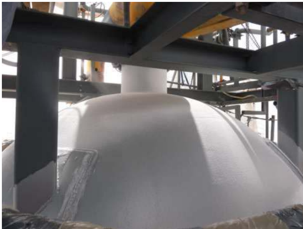
First layer of HOT SURFACE COATING at 1,5 mm
