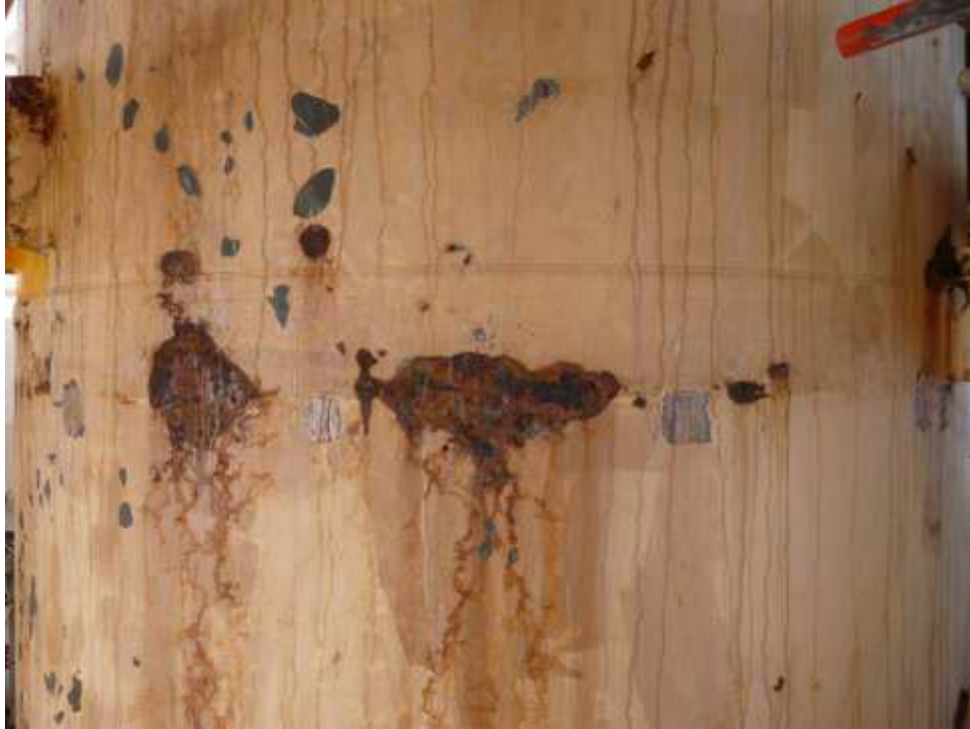
Vessel after removing the insulation material
