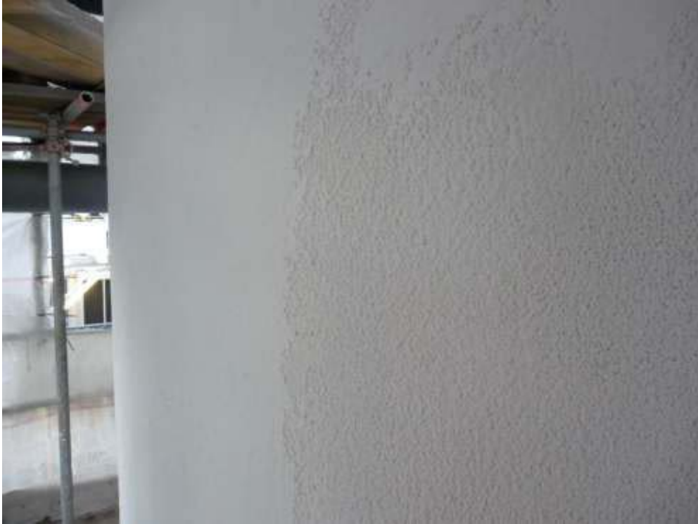
Surface partly troweled (left)
