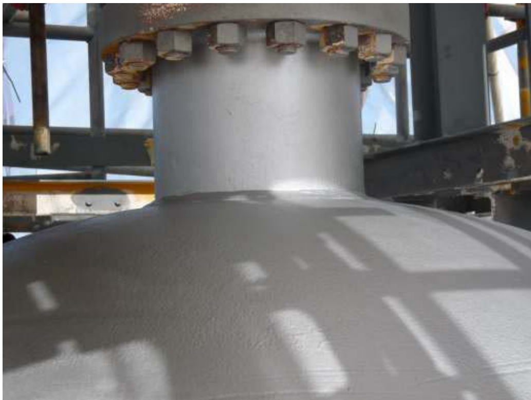
Top completed with RUST GRIP
