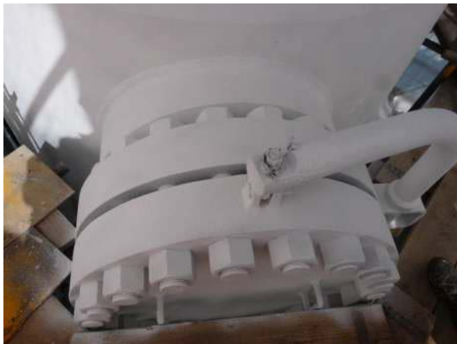
HOT SURFACE COATING applied on manhole
