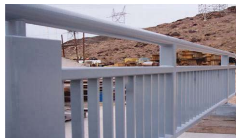
Railings were power washed at 3,500 psi and primed with Rust Grip®.
