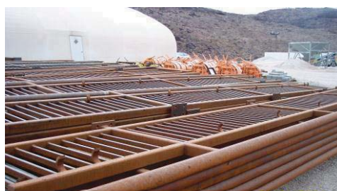
Steel railings were allowed to develop flash rust in preparation for the Rust Grip® application.
