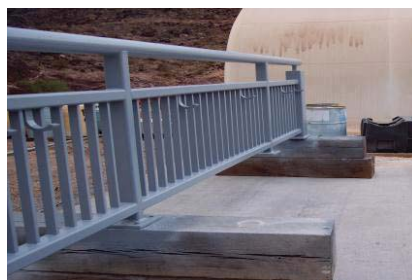
Steel railings were allowed to develop flash rust in preparation for the Rust Grip® application.
