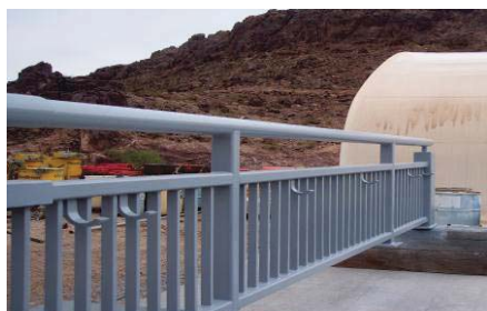
Railings were power washed at 3,500 psi and primed with Rust Grip®.
