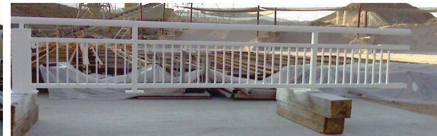
Super Therm® was applied to prevent heat from loading onto the steel railings, possibly burning visitors.
