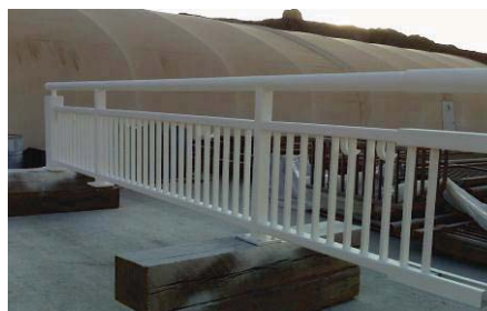
Super Therm® was applied to prevent heat from loading onto the steel railings, possibly burning visitors.
