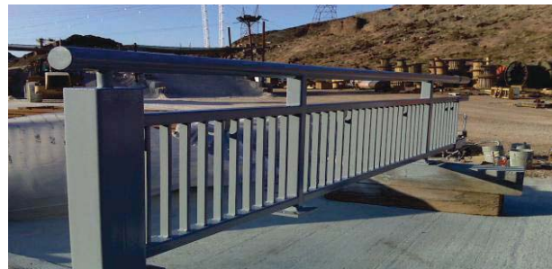
Enamo Grip topcoated Super Therm® to prevent hand oils from deteriorating surface.
