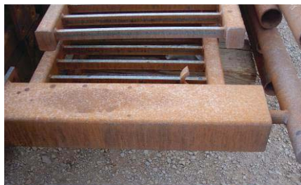
Steel railings were allowed to develop flash rust in preparation for the Rust Grip® application.
