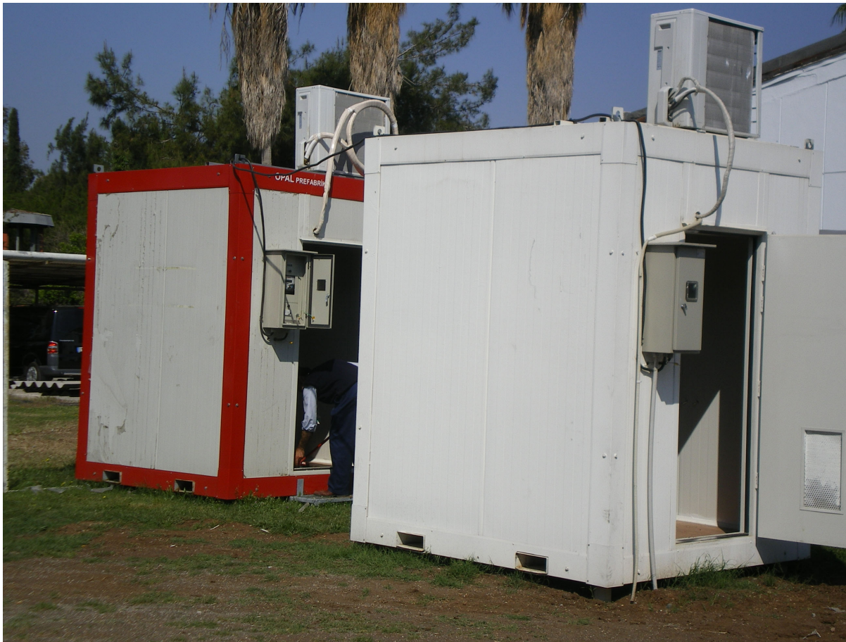
Both shelters at test facility of Vodafone, Adana, Turkey
