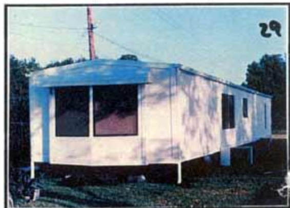
Mobile home when painted on roof and sides reduced its utility consumption by as much as 60%.
