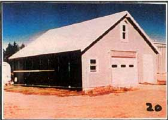
One of the manufacturing buildings located at Ag Enterprises in Grainfield, Kansas coated with SUPER THERM. The upper floor dropped 24 degrees and bottom floor dropped 12 degrees over the span of the entire summer period.
