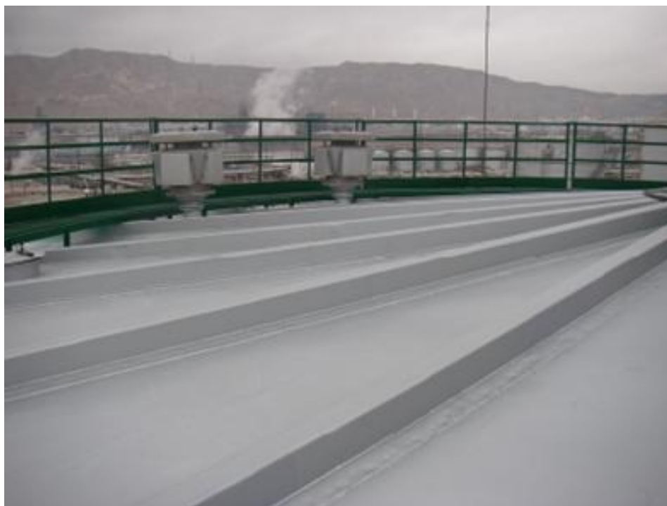
Tank finished with Rust Grip®
