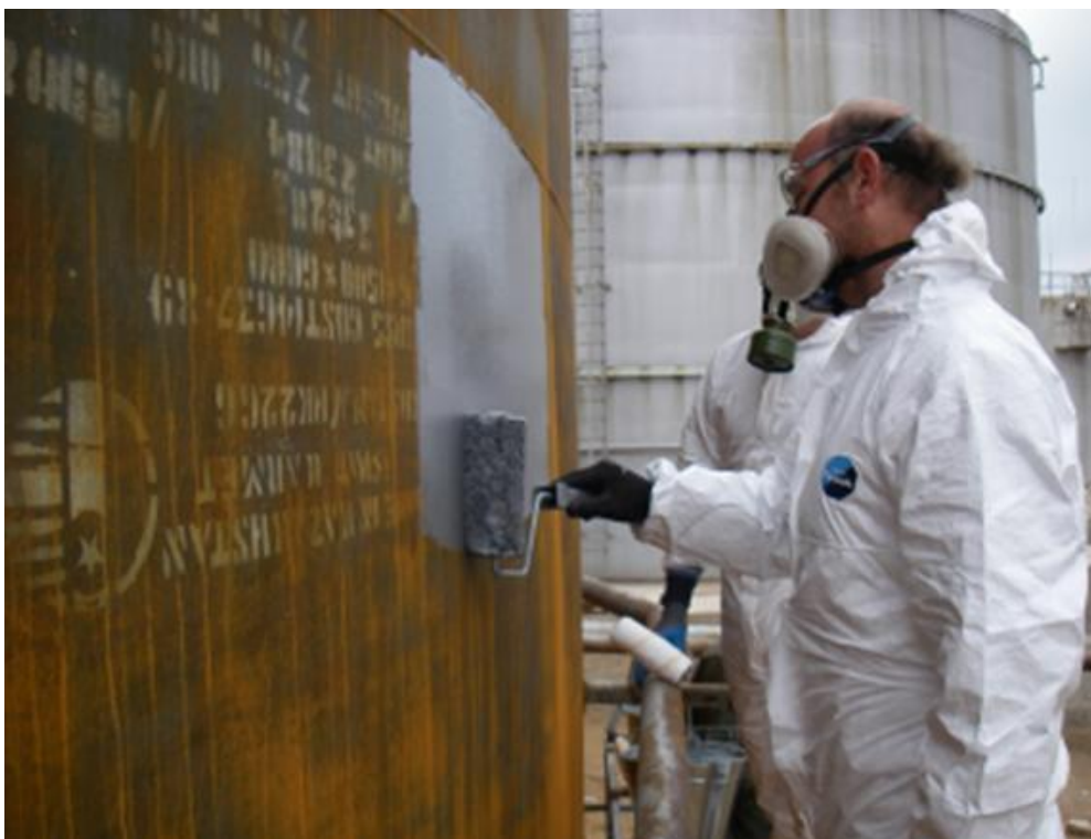
Rust Grip® was applied by roller. No Acetone was available but the surface was dry and clean.
