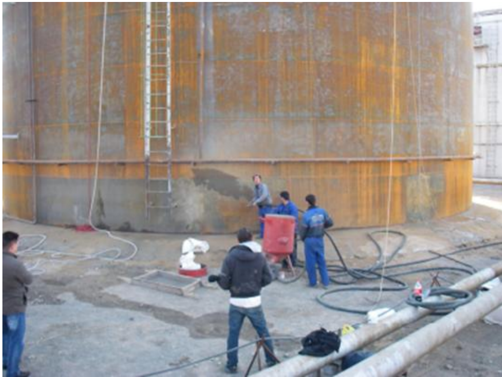
Removing of the old coating and mill scale by water sand blasting.
