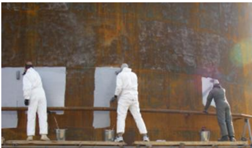
Application of first layer Rust Grip® at 125µ WFT by roller.
