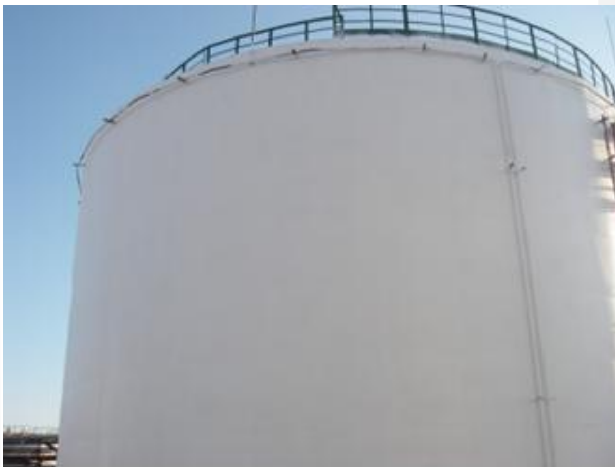
Finished tank with Super Therm®
