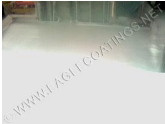
Bottom Floor with Electric Heater ( DRY HEAT ) to speed up the cure down. Bottom Floor clean, dry and sound ready to accept a coating of SUNSHIELD ®
