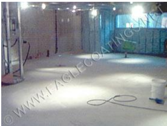
All 3 floors where completed in 1 day by sealing all openings and applying Electric heat. Installation of the radiant heating system was started the next day on schedule.
