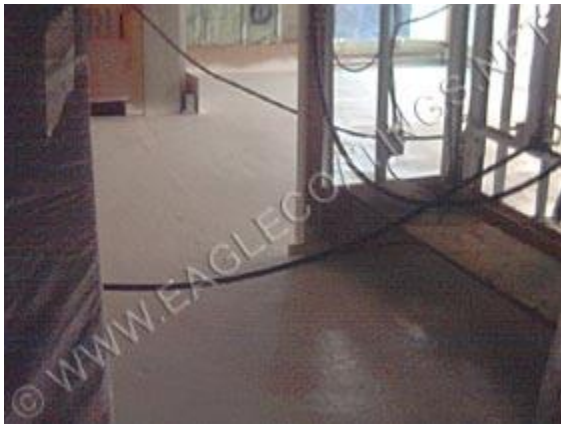
Bottom Floor with Electric Heater ( DRY HEAT ) to speed up the cure down. Bottom Floor clean, dry and sound ready to accept a coating of SUNSHIELD ®
