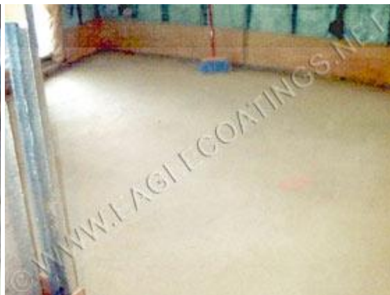
All 3 floors where completed in 1 day by sealing all openings and applying Electric heat. Installation of the radiant heating system was started the next day on schedule.
