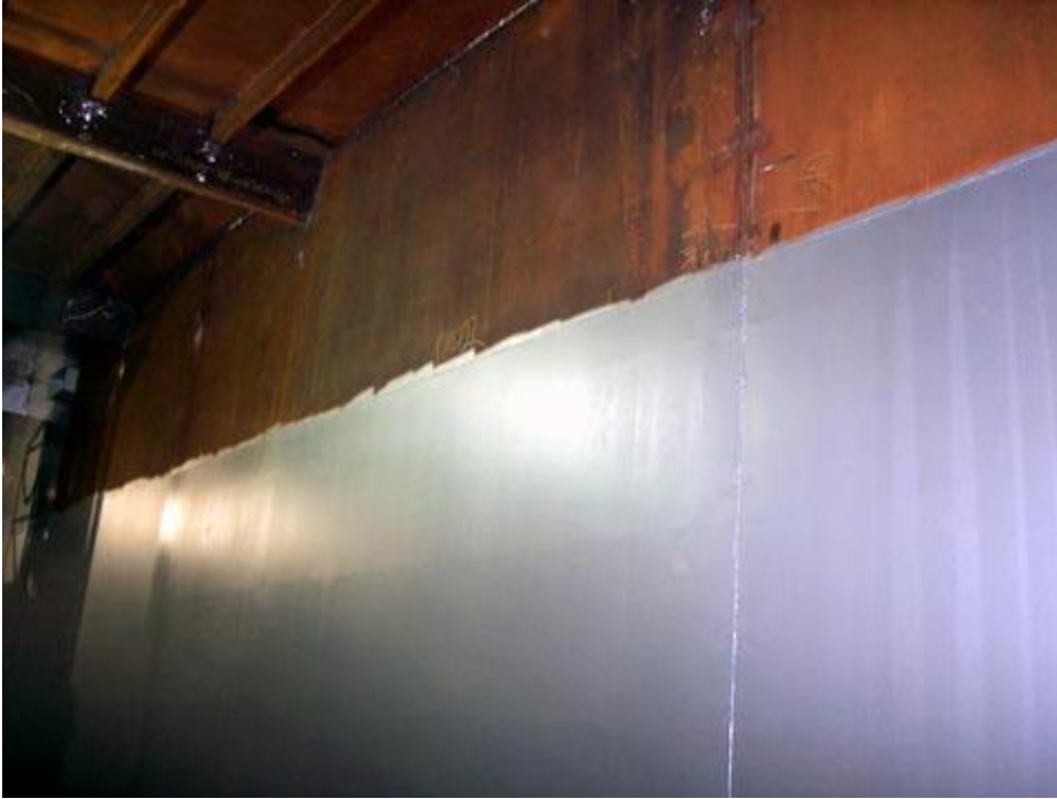
Inside the Ballast Tanks
