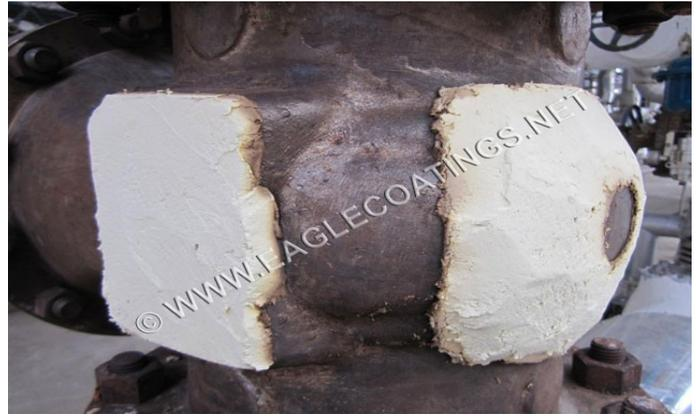
The coating was applied at a thickness of 7mm (276mils) - 10 mm (394 mils) DFT
