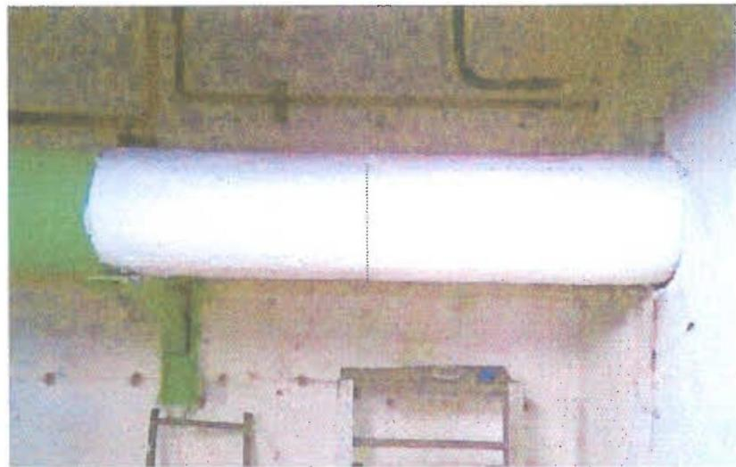
Afterwards pipe surface temperature 6,4°C with condensation,
