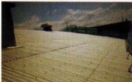
Application of SUPERBASE
