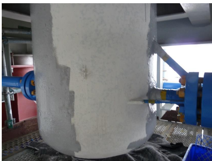
First layer of EnduRoof applied on V-1137
