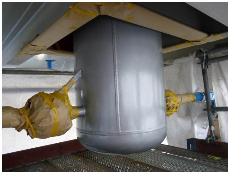
V-1137 after applying Rust Grip
