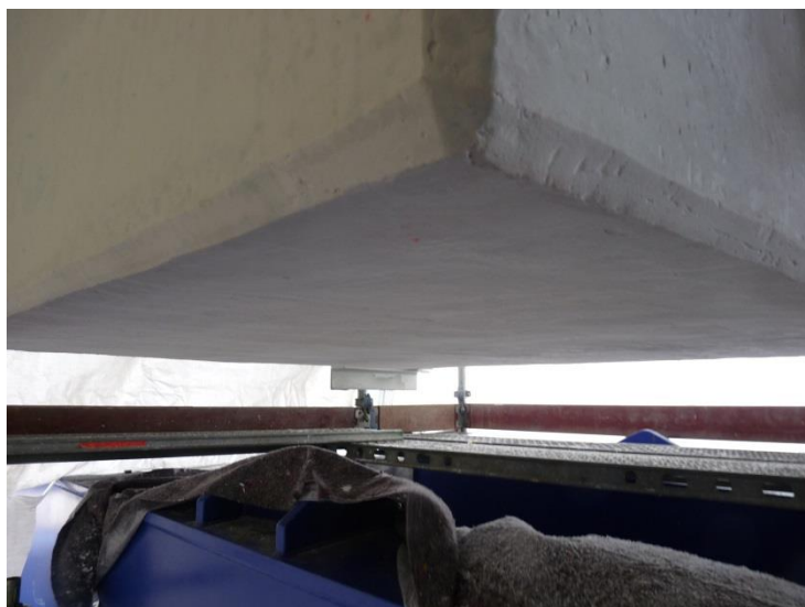
Surface smoothened by stuccoing and sanding
