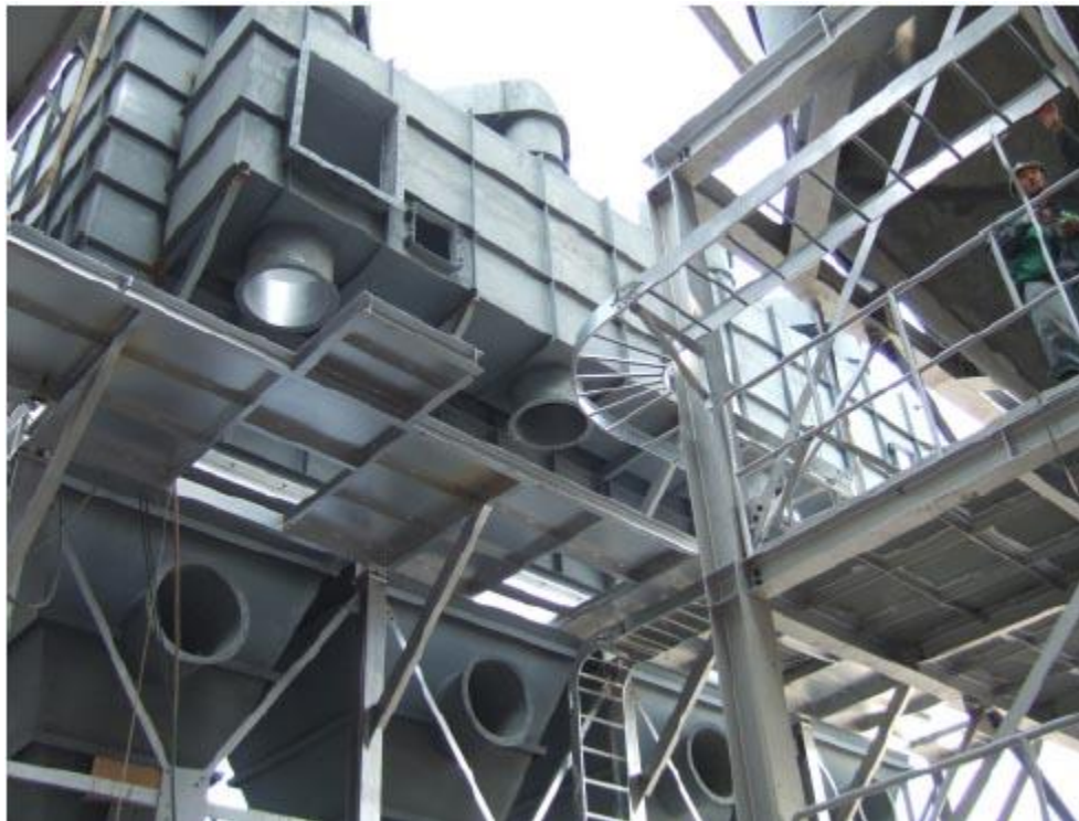
Filtration Interior facility after coating
