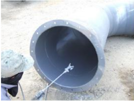
2nd application of RustGripRustGrip after 2nd coating
