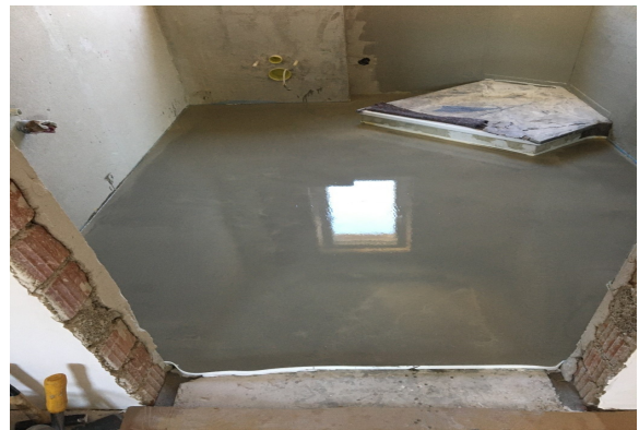
Filled underfloor heating
