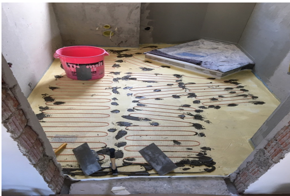
Insert and fix the heating loops
