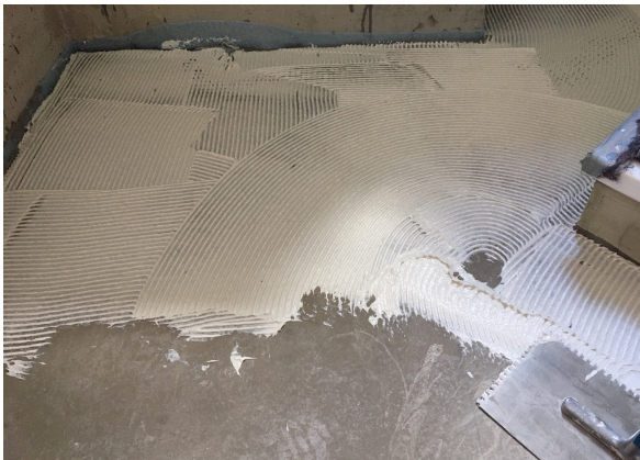
Coating minimum 1 mm HPC (filler)
