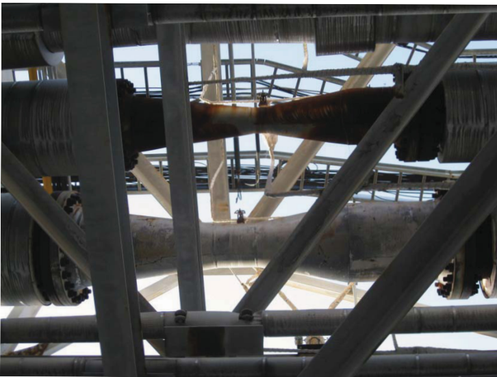
Flange Before coating: 160^{\circ}\text{C}
