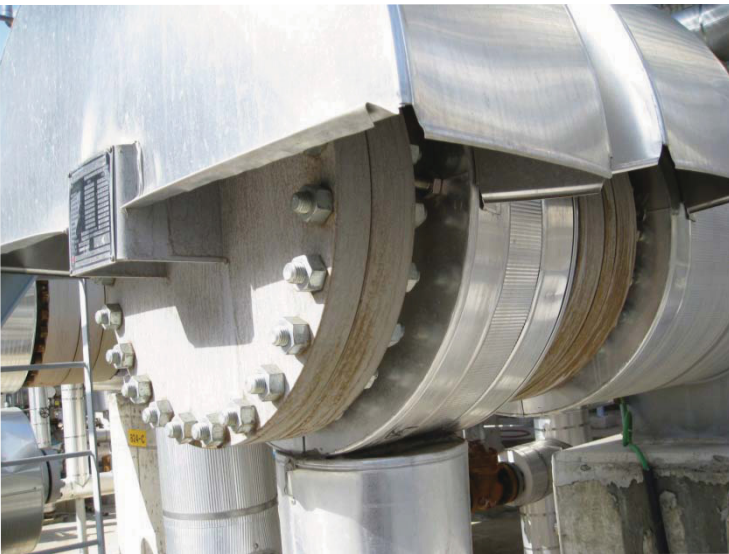
Flange Before coating: 130^{\circ}\text{C}
