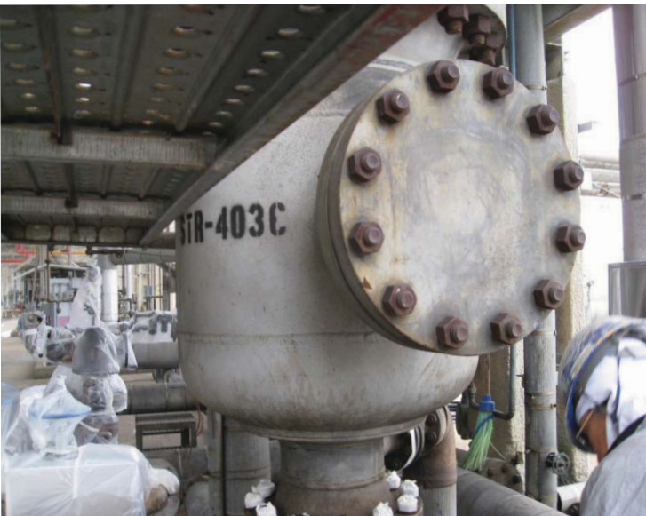
Strainer Before coating: 170^{\circ}\text{C}
