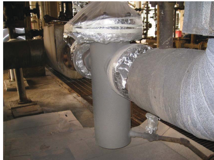
Strainer After coating: 50^{\circ}\text{C}
