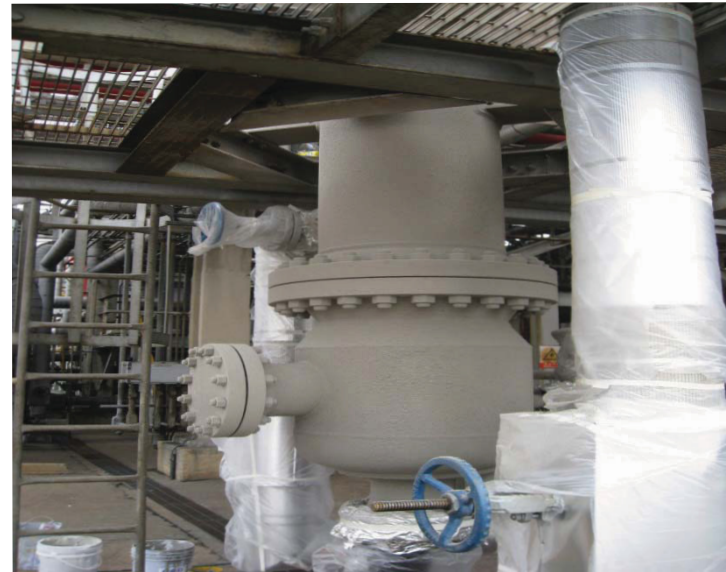
Strainer After coating: 45^{\circ}\text{C}
