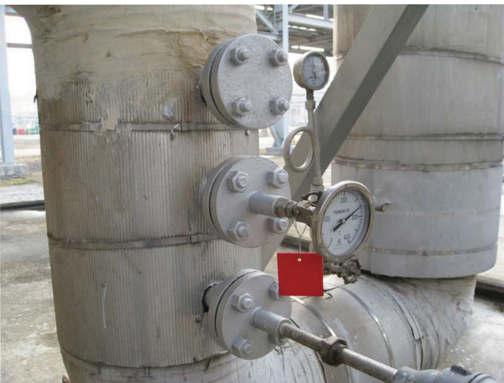
Flange Before coating: 130^{\circ}\text{C}
