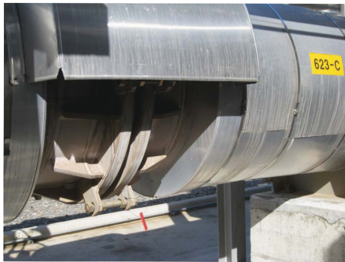
Flange Before coating: 130^{\circ}\text{C}
