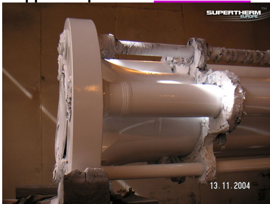
Applied top coat of ENAMO GRIP ®
