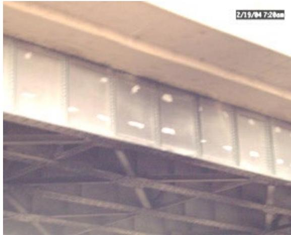
**Problem: Trains operating under the bridge leave severe diesel soot and carbon deposits behind, resulting in a corroded bridge structure.**
