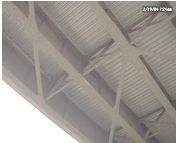
**Solution: Two coats of RUST GRIP ® applied by brush at 200 sq.ft.(18 sq. meters) per gallon, covered by ENAMOGRIp ® sprayed on using an airless sprayer at 250 sq.ft.(22 sq. meters) per gallon. Tip size was .016 (16/1000 inch) or 400 micron (0.4mm).**
